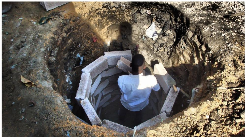
**Appendix 1—figure 6.** Construction of a soakaway pit for discharge of liquid effluent from intervention latrines.
